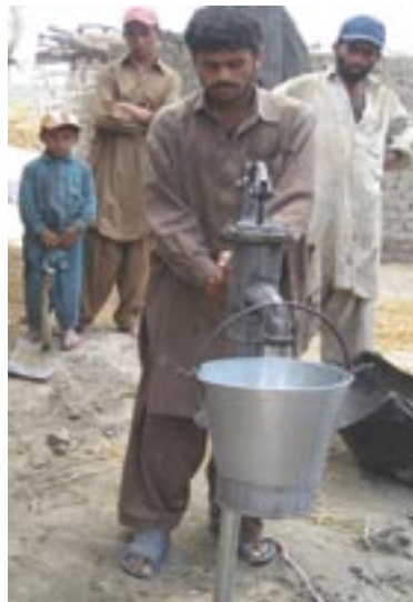
Water Hand Pump Installed in a Village
